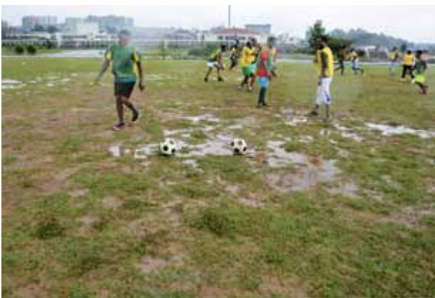
a) Poor drainage leading to loss of grass cover.
