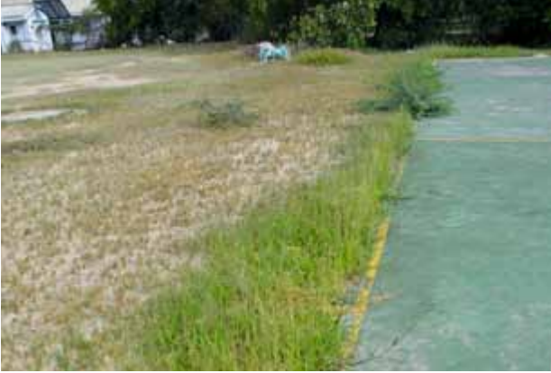
a) Unwanted vegetation around the sports ground due to lack of regular cleaning and mowing .
