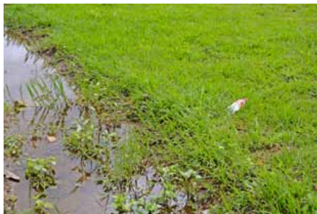
b) Poor surface levels, poor drainage and weed invasion.
