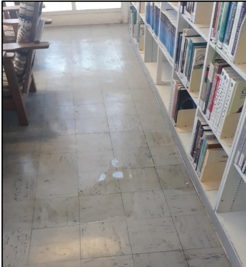
The sewage water leakages at the Katutura Intermediate Hospital library.
