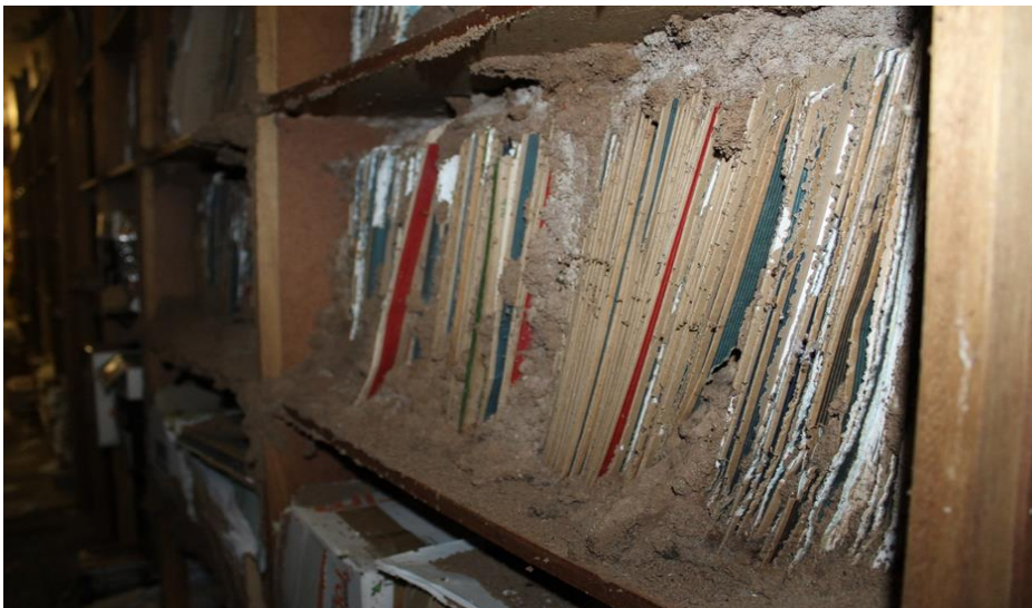
Records damaged by termites inside a Records Centre: Picture taken in January 2018
